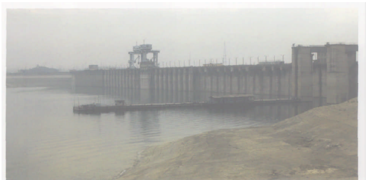
The giant dam at the outlet of the Danjiangkou Reservoir.
